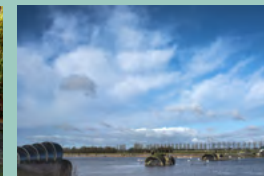
The 'balgstuw' (inflatable dam) near Ramspol protects against high tides from the Ketelmeer (p 38)
