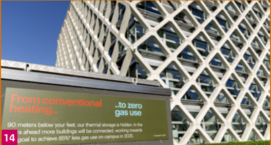
14 At the Wageningen University Campus, buildings are being connected to the hot and cold storage (ATES) system. This sustainable energy system will allow the university to reduce approximately 75% of its natural gas use by 2025 compared to 2019. Flexibility in building as well as making existing buildings sustainable are key to meeting the climate goals. (p. 27)
